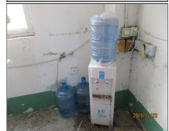
External photo(s) of the production unit(s) Water-Drinking Area.JPG
